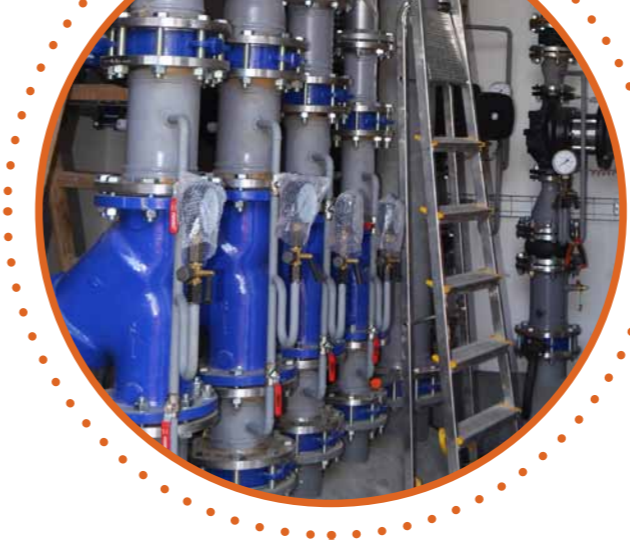
COOLING MACHINE ROOM
