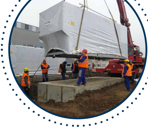
MOVING OF CHILLERS TRANSFORMER STATION
