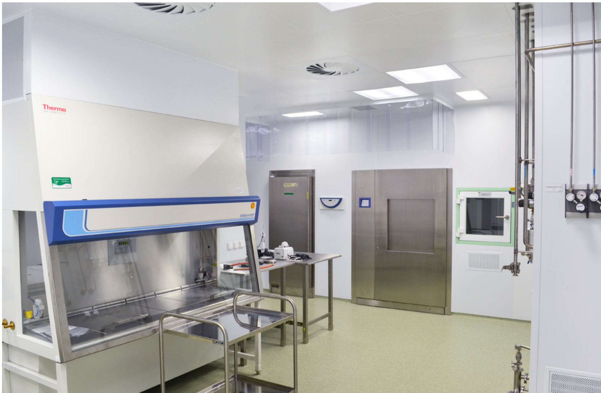
Building A - Research laboratories
