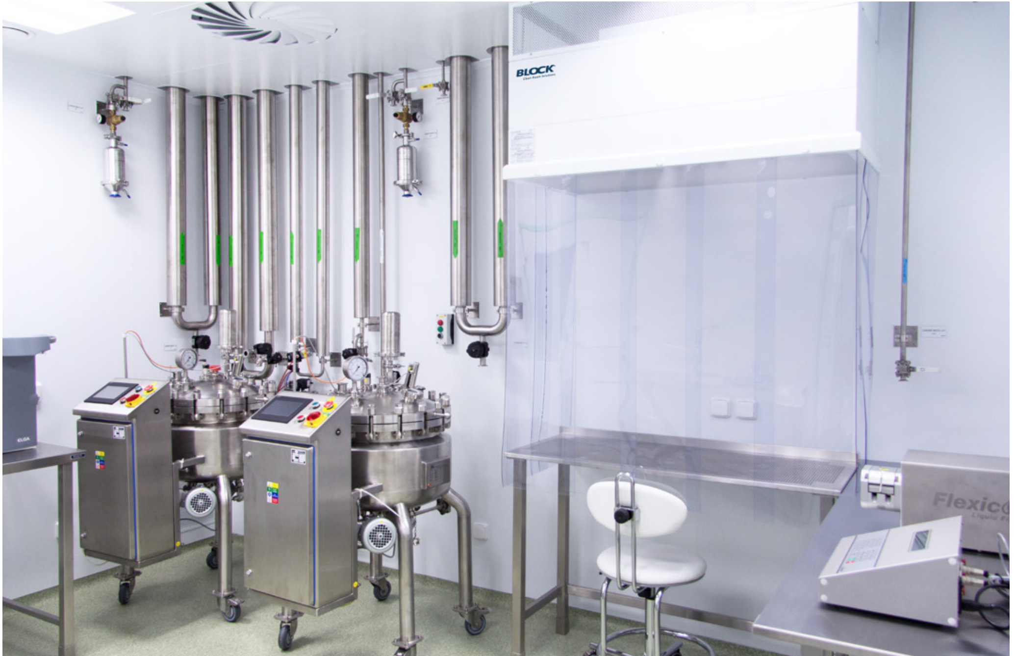
Building A - Research laboratories
