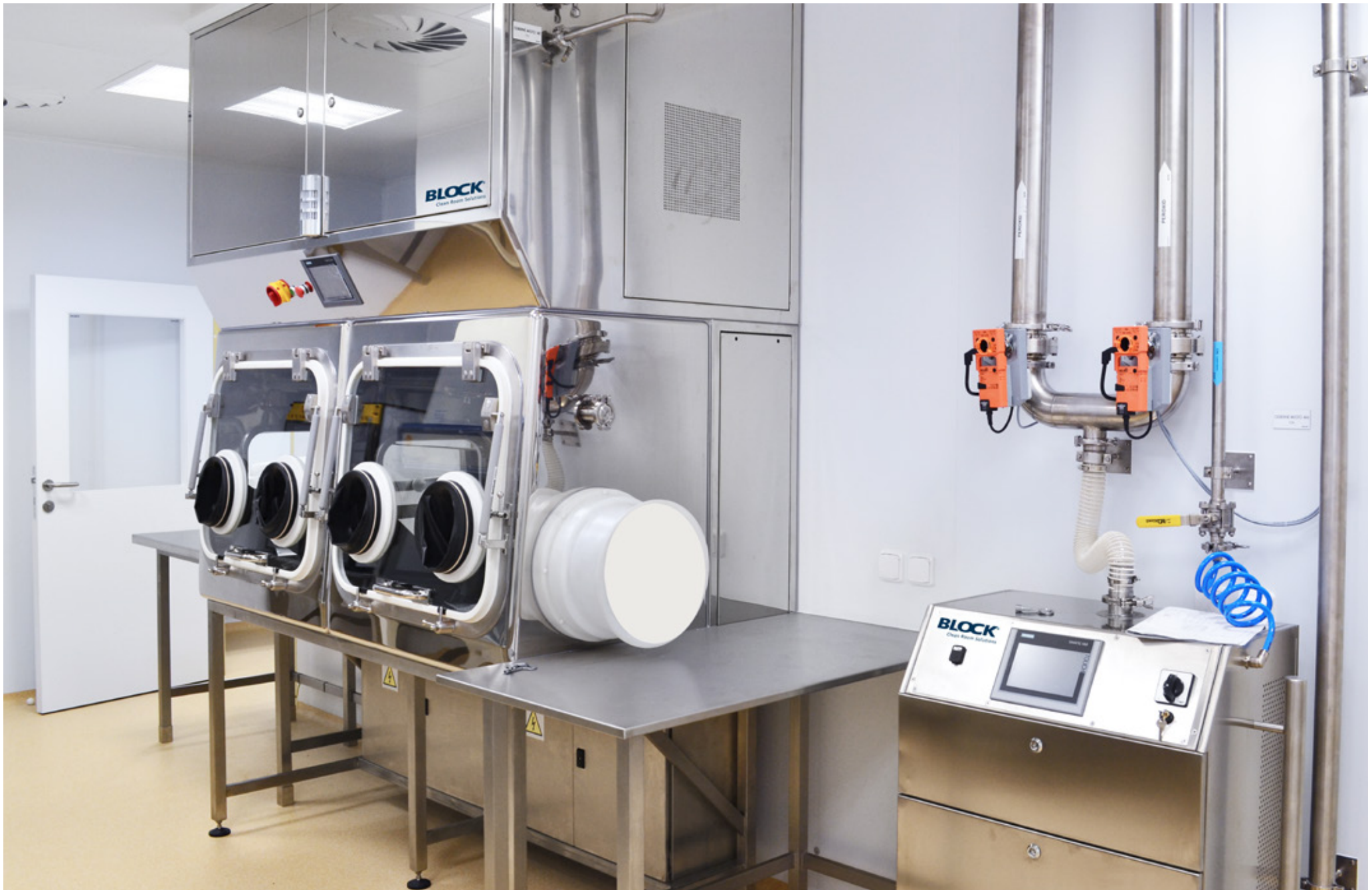
Building A - Research laboratories
