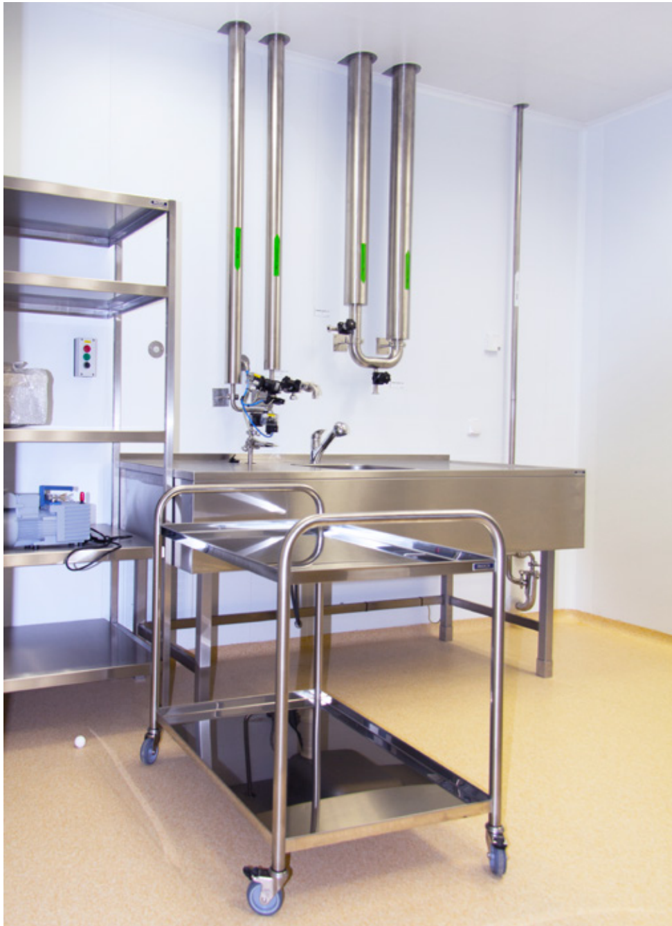
Building A - Research laboratories
