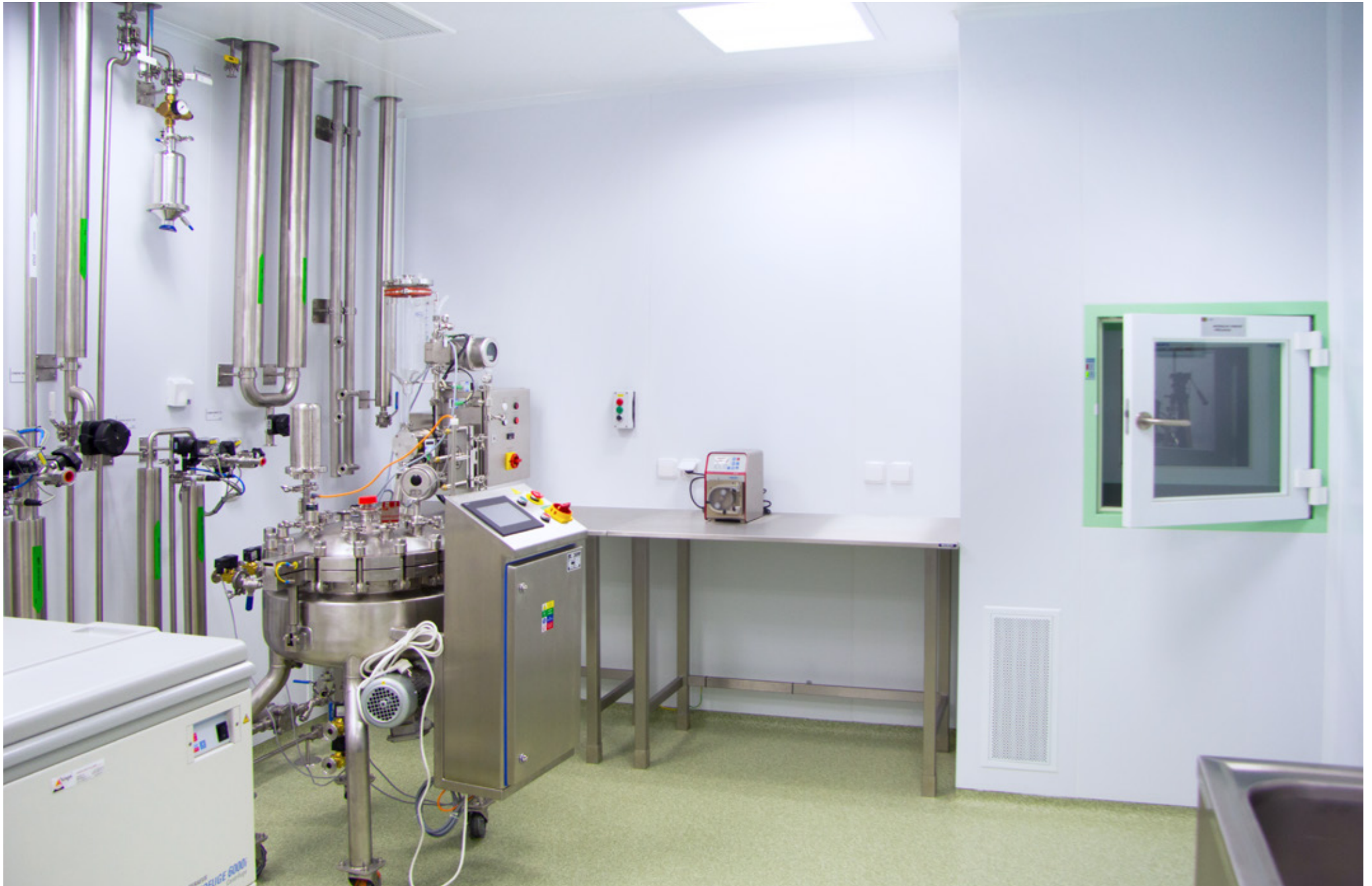
Building A - Research laboratories
