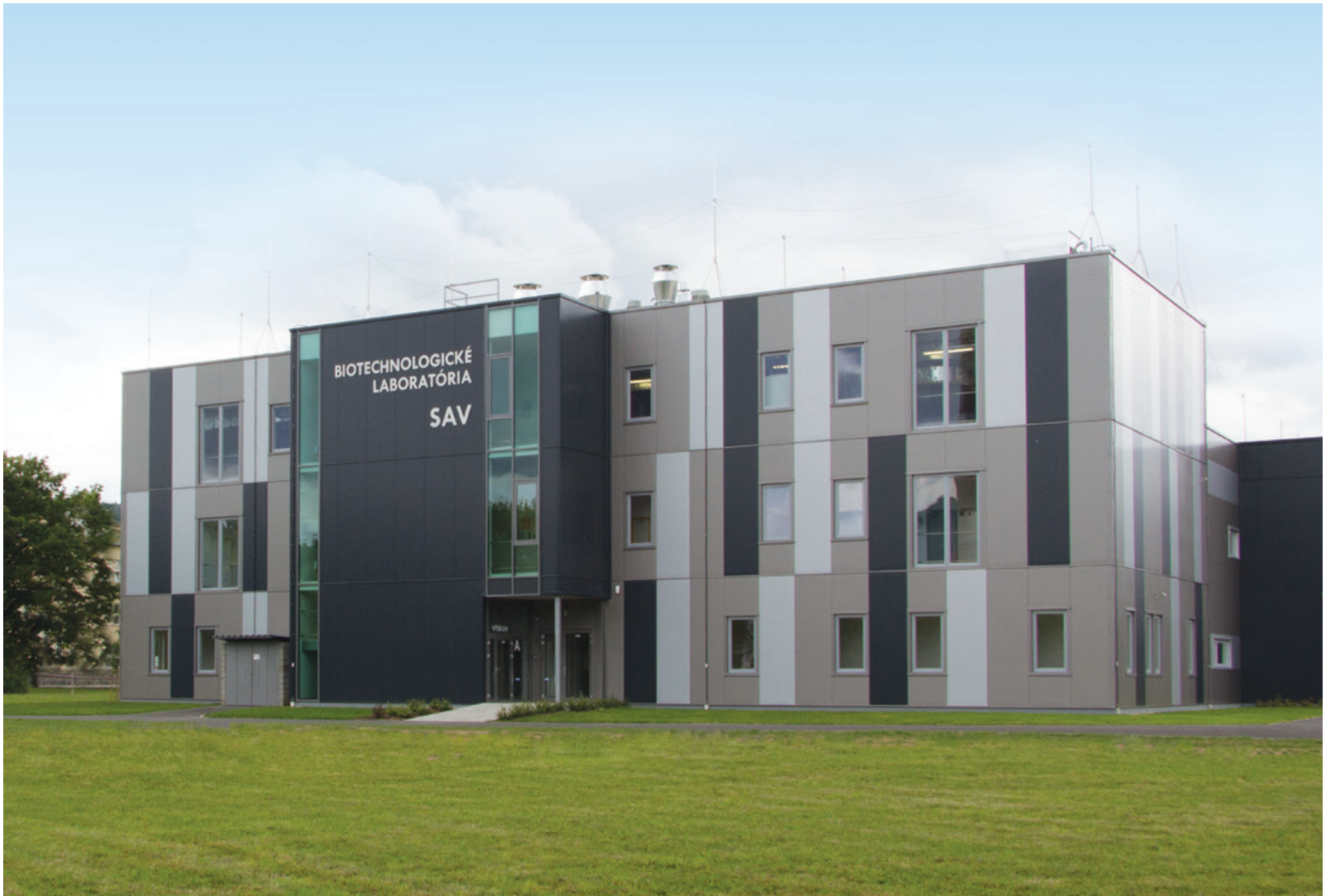
Build-up of the R & D Centre of Immunoactive Substances | Slovak Academy of Sciences | Šarišské Michaľany; Slovakia | 2015
