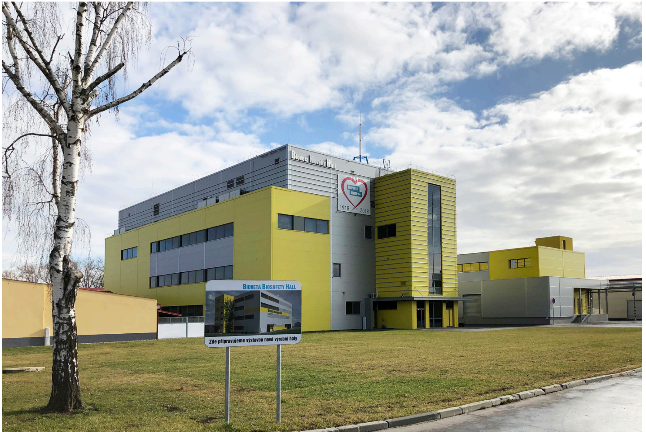
Virology Department on the 2nd Storey Above Ground of The Bioveta Novelty Hall (BNH) | Bioveta a.s, Ivanovice na Hané | Czech Republic | 2018
