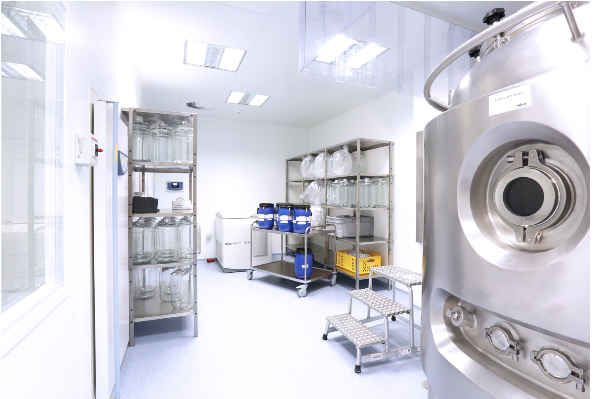
Virology Department on the 2nd Storey Above Ground of The Bioveta Novelty Hall (BNH) | Bioveta a.s, Ivanovice na Hané | Czech Republic | 2018
