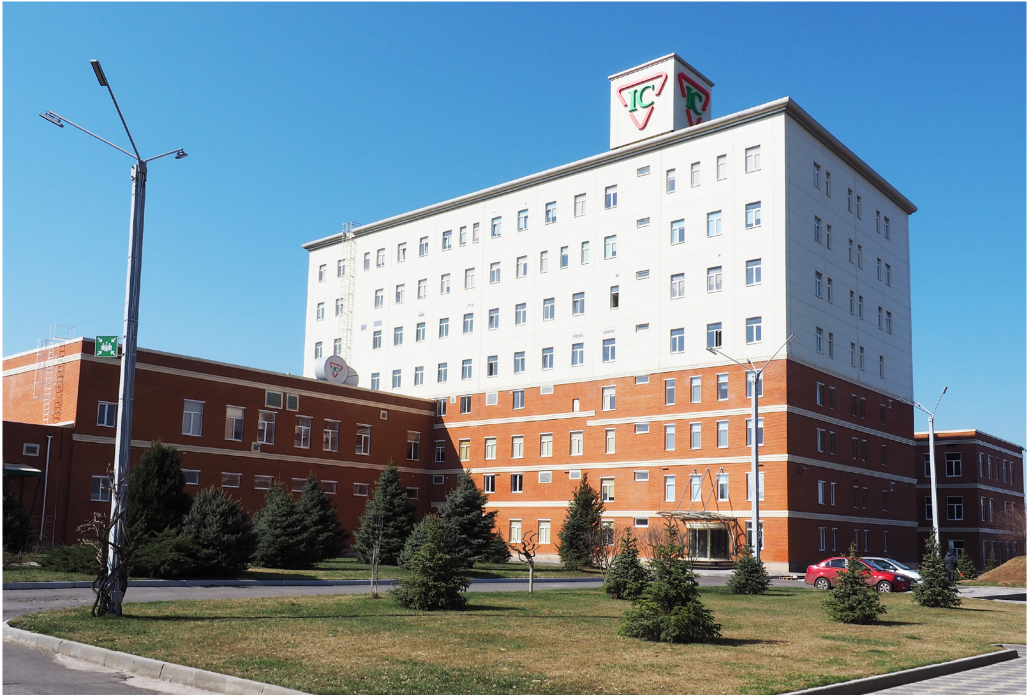
Construction of a Facility for the Production of Substances, GLS Production and Administrative Laboratory Complex | InterChem | Ukraine | 2015
