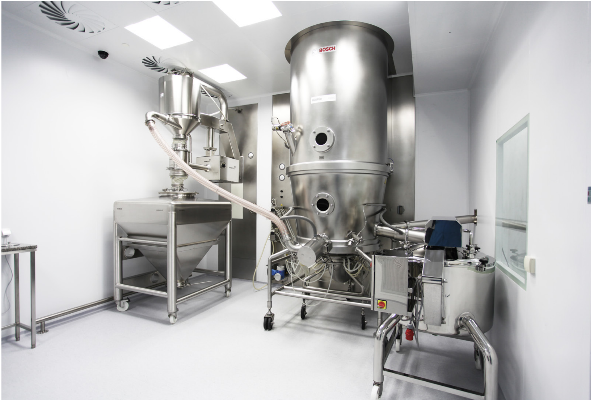
Construction of a Facility for the Production of Substances, GLS Production and Administrative Laboratory Complex | InterChem | Ukraine | 2015
