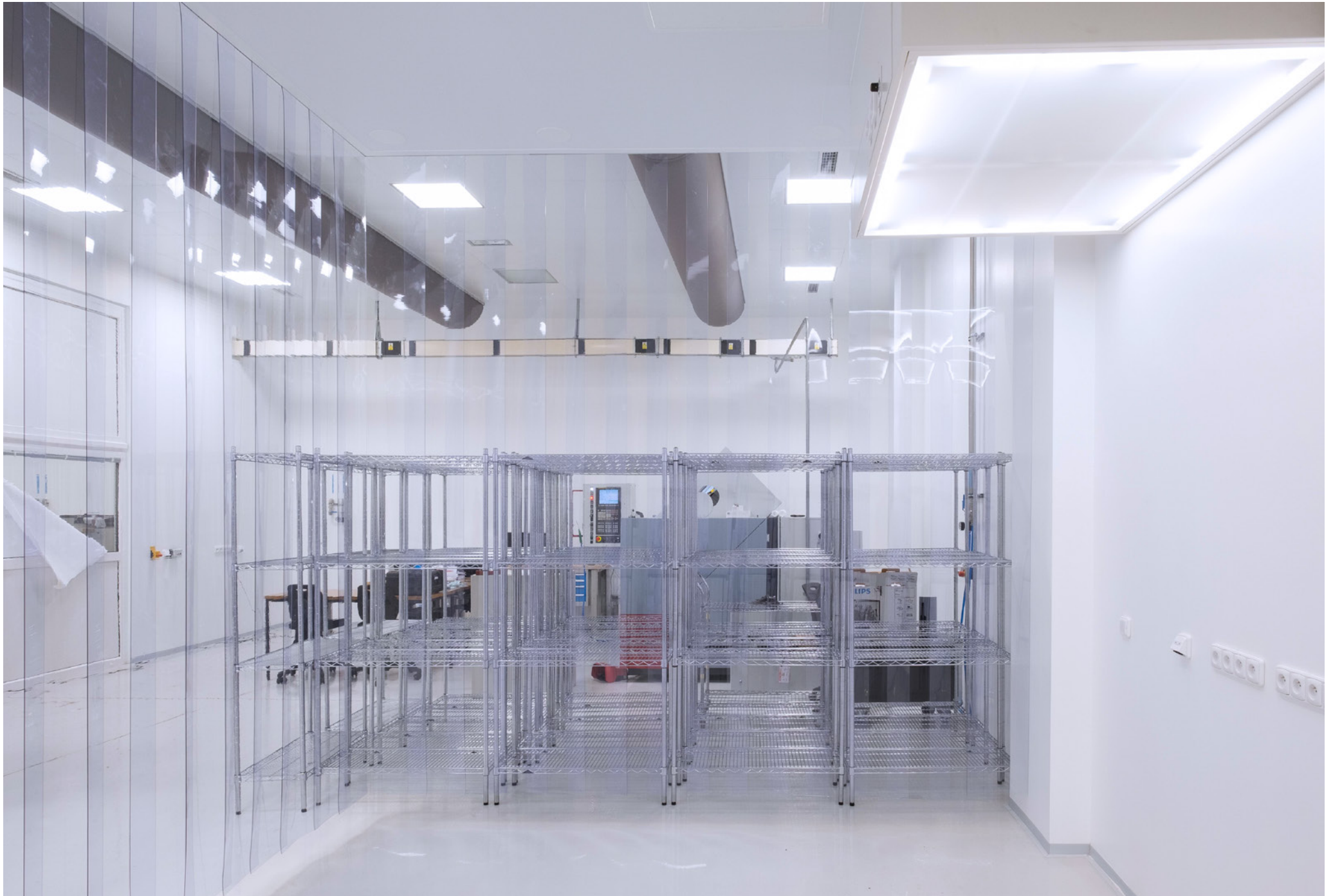
Construction work rooms for precise machining of components | Meopta - optika, s.r.o. | Přerov, Czech Republic | 2016
