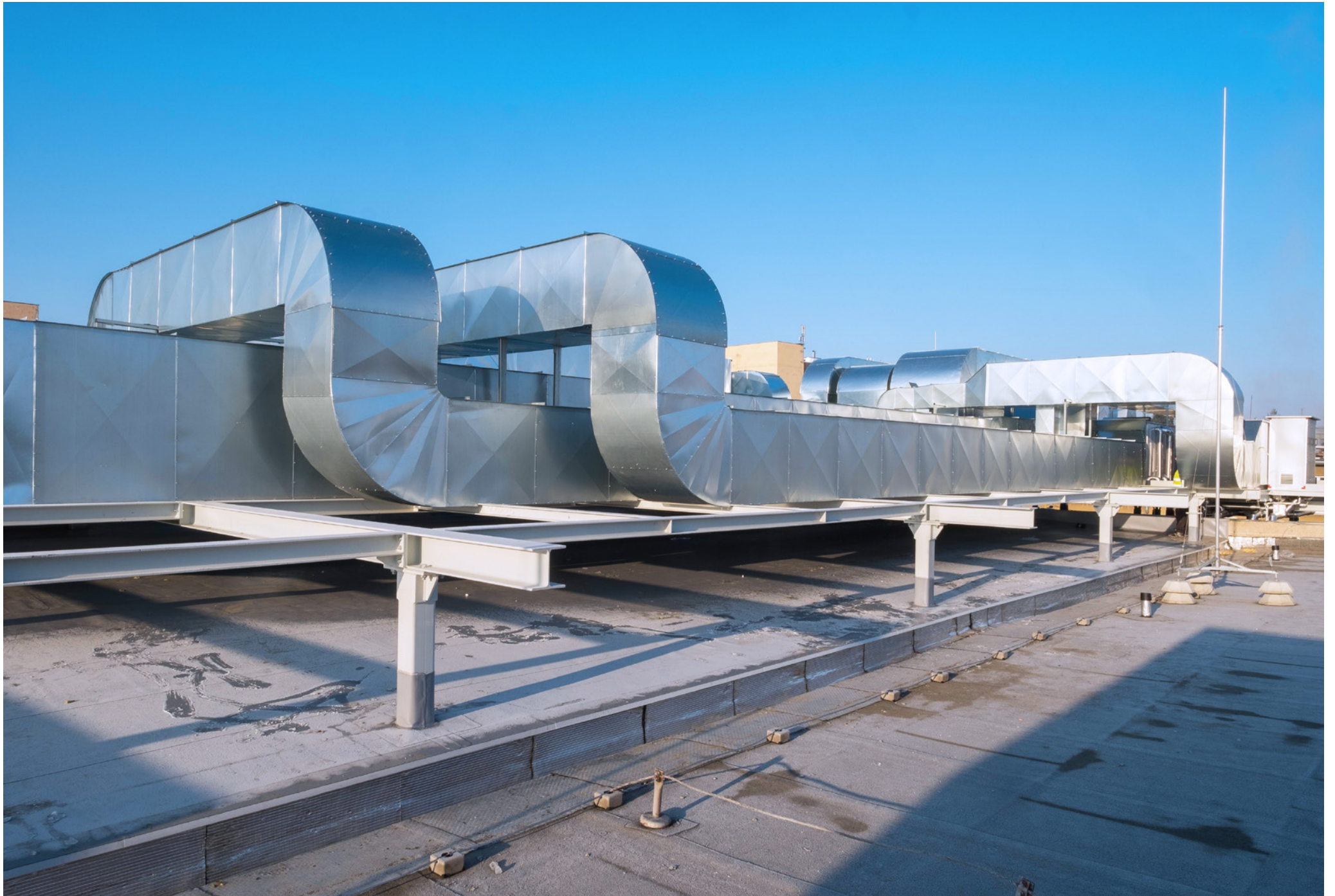
Construction work rooms for precise machining of components | Meopta - optika, s.r.o. | Přerov, Czech Republic | 2016
