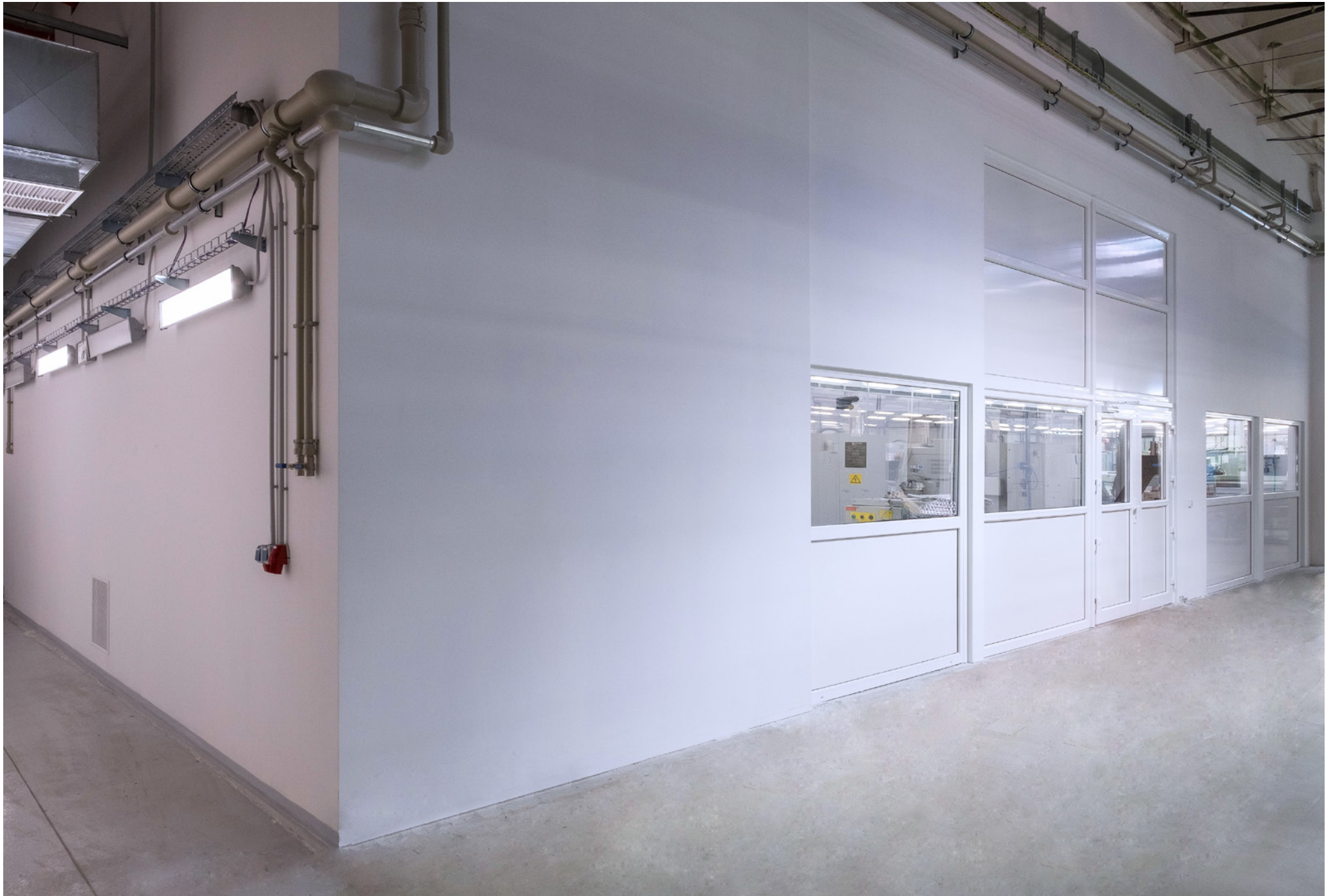
Construction work rooms for precise machining of components | Meopta - optika, s.r.o. | Přerov, Czech Republic | 2016
