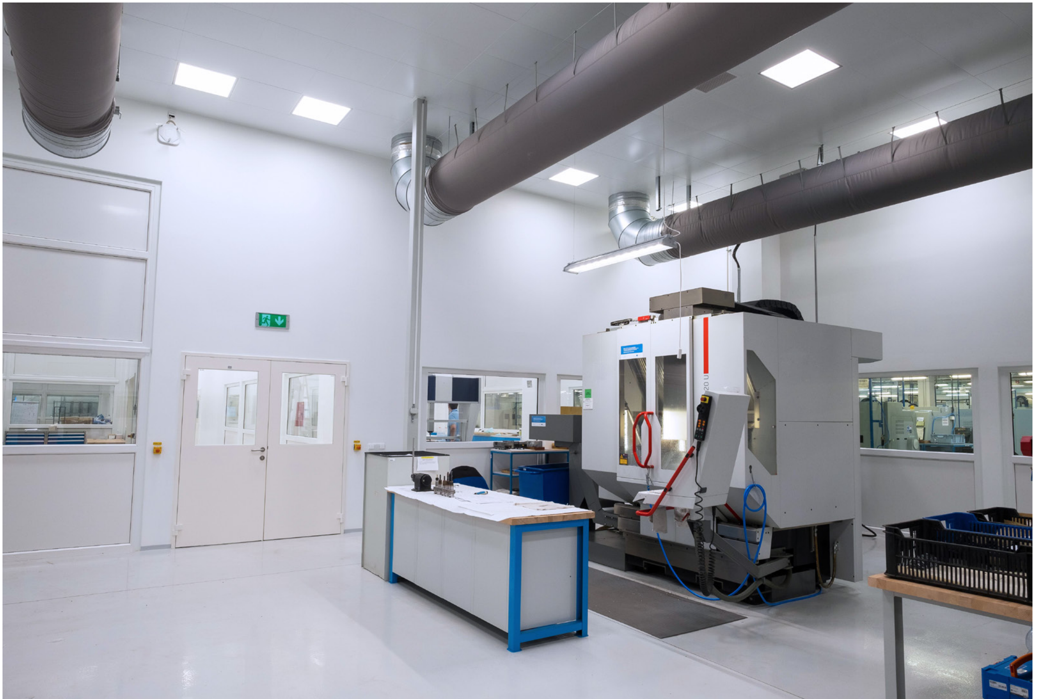
Construction work rooms for precise machining of components | Meopta - optika, s.r.o. | Přerov, Czech Republic | 2016
