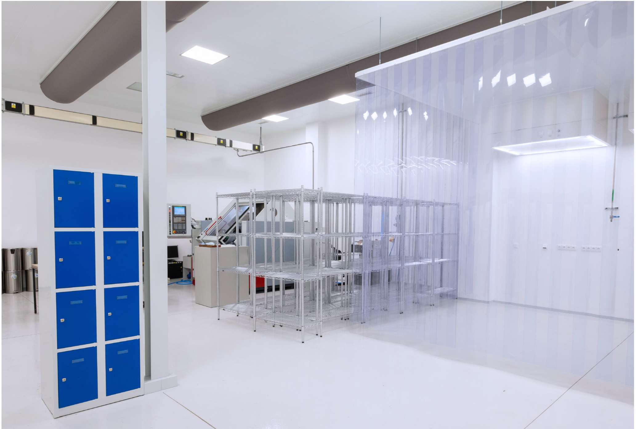
Construction work rooms for precise machining of components | Meopta - optika, s.r.o. | Přerov, Czech Republic | 2016
