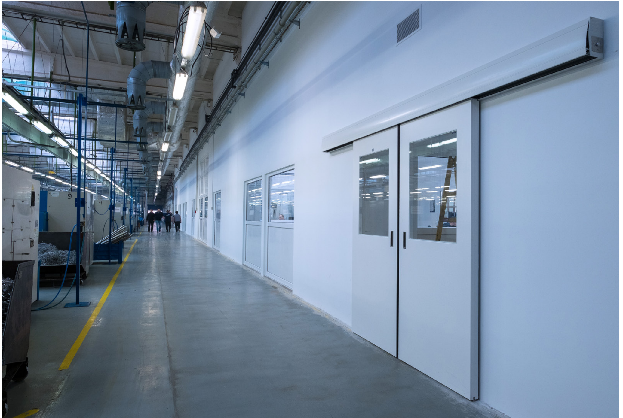
Construction work rooms for precise machining of components | Meopta - optika, s.r.o. | Přerov, Czech Republic | 2016
